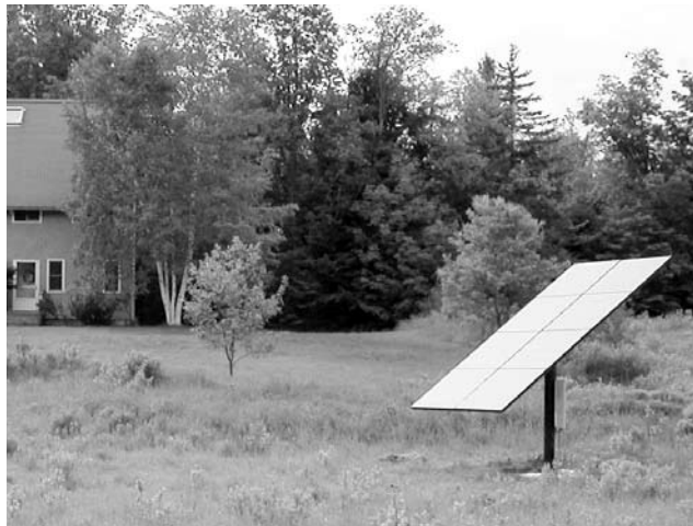
A small solar array in the yard can produce half of this homeowner's power.
