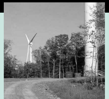
Wind power is becoming a reality in Vermont. Shown here is the completed and restored access road at the Sheffield Wind site, with Turbine #4 in the foreground and Turbine #6 in the rear. The turbines will turn for real in Sheffield next month. Story, page 3.
