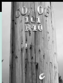
Utility poles tell a story if you know what you're looking for – whose pole it is, location indices, what birds, animals and insects have passed by. The pole-inspection story continues on page 8.
