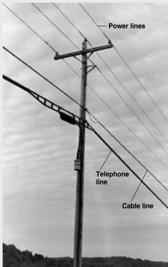
Knowing what's on a utility pole helps you know which company to call if you see trouble. But most important is that you call someone .
