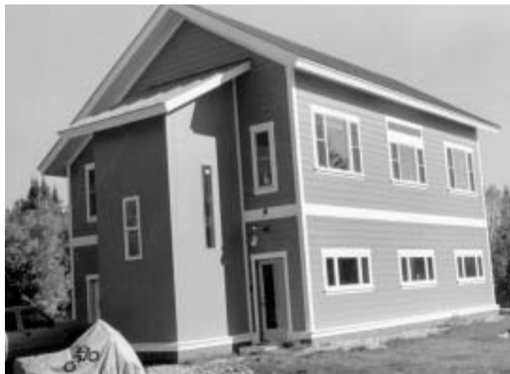
Robert Henderson's Williamstown home, constructed with Structurally Insulated Panels, was the most energy-efficient house built in Vermont in 2002.
