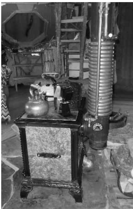
Author Steve Miller's Hearthstone wood stove, with a heat exchanger coiled around the vertical stove pipe.
