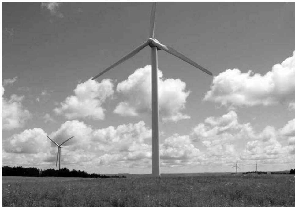
Wind farms and methane power plants are cropping up around New York State as electric co-ops and other utilities combat rising power costs with local, renewable energy. Pictured above is the Fenner Wind Farm in Morrisville; unfortunately, the local co-op can't tap into its power, but at least the wind farm is greening up the New York grid.
