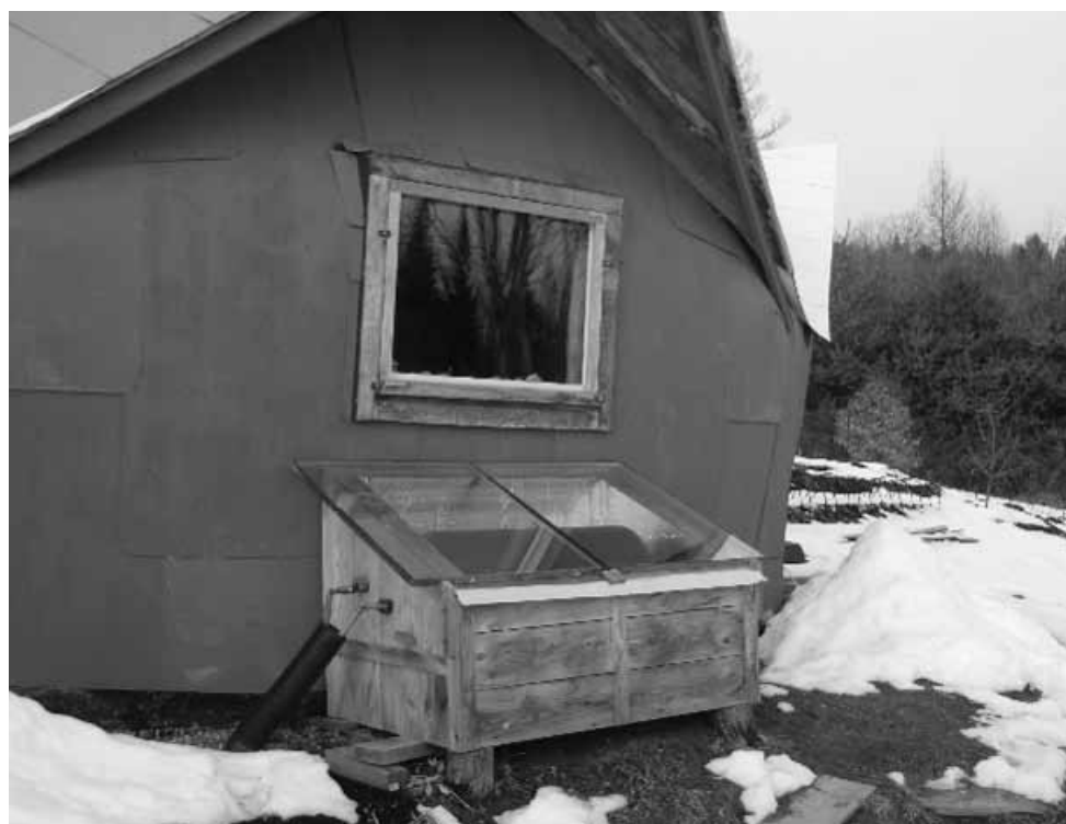
Low-tech solar water heating at work. An old stripped-down water tank inside this glass-covered box captures the sun's energy and pre-heats the family's domestic hot water.
