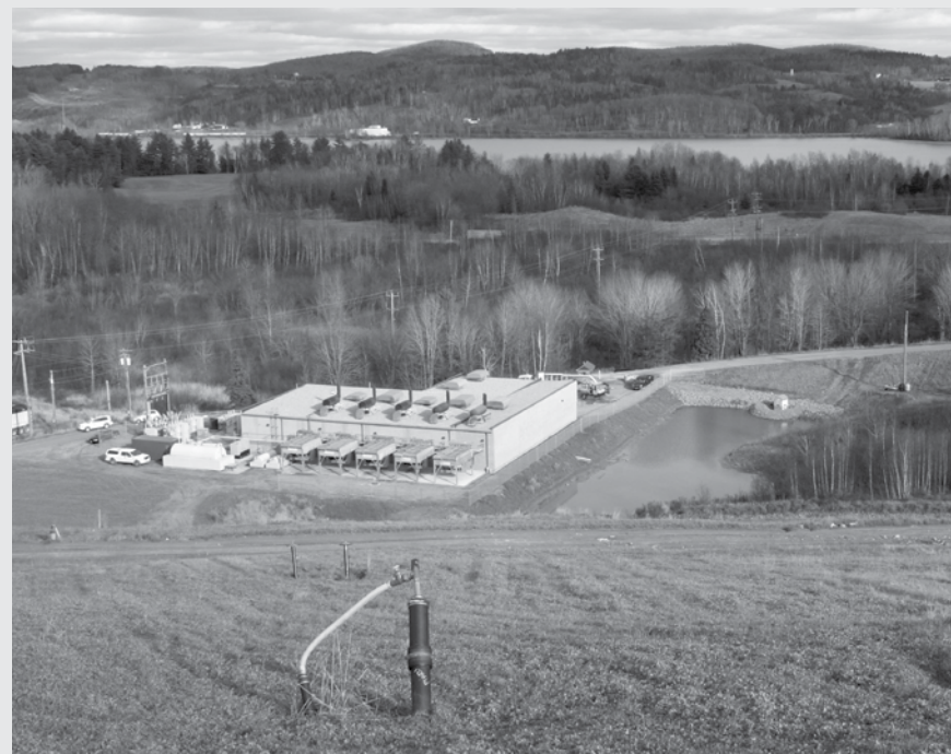
Arguably, the most significant undertaking by the Co-op's Board in this decade was the construction of the Coventry, Vermont, electric-generating station, seen here from atop the landfill that produces the methane that fuels the power-producing engines. Opened in 2005 and expanded in 2009, the plant produces an ever-growing portion of WEC's energy (now exceeding half, and increasing), at below-market rates.
